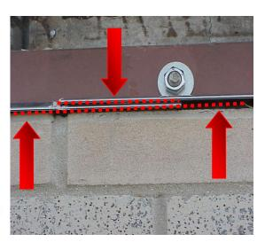
Also, we should be installing a silicone sealant, such as Dow 790, under the stainless steel flashing and just under the hemmed edge & the face of the masonry in order to make sure that water does not enter the system below the wall flashing.
