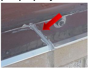
We should be installing a silicone, such as Dow 790, at the splice, located at all sides (Box Pattern), and at the front of the drip edge.
